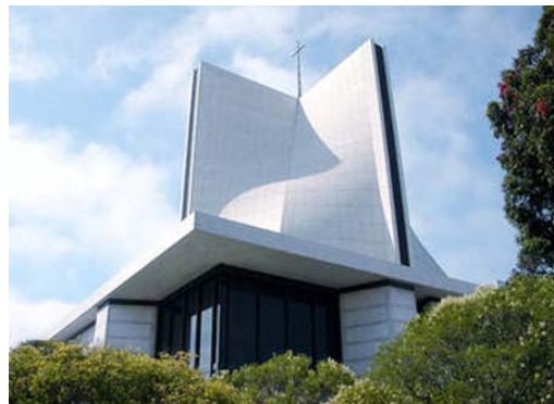
Figure 8. Cathedral of Saint Mary of the Assumption in San Francisco, RC roof structure by P.L.Nervi
