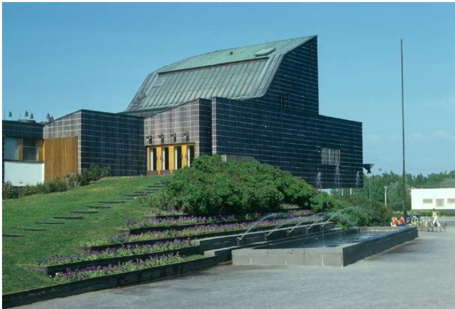
Figure 6. Hall Twon in Seinäjoki (Alvar Aalto, 1958). Source: http://larryspeck.com/2011/02/02/seinajoki-town-hall/
