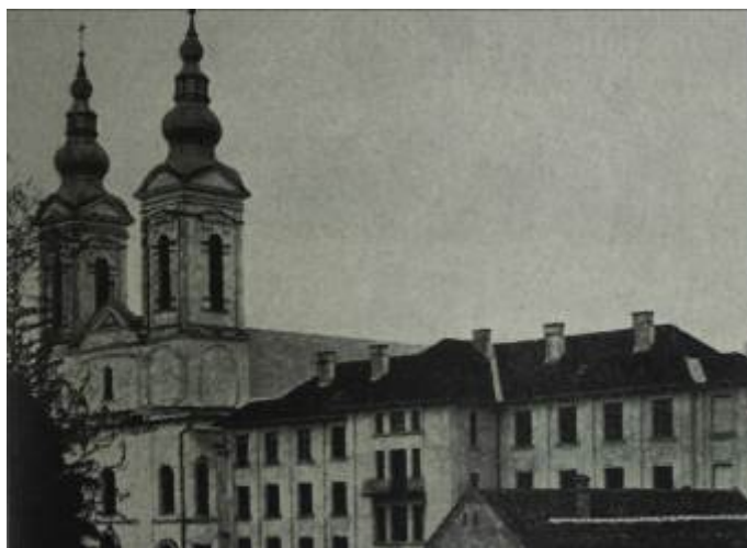
Figure 3. The Church and the Second Convent of the Assumption of Mary: view from the west; photograph taken in 1930 [5]
